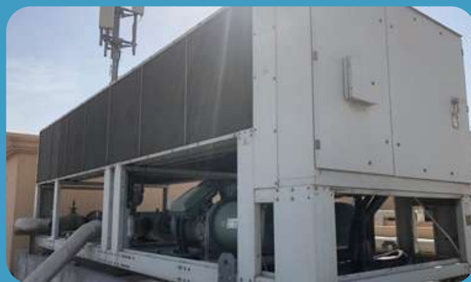
> Chiller Installation & Replacement
